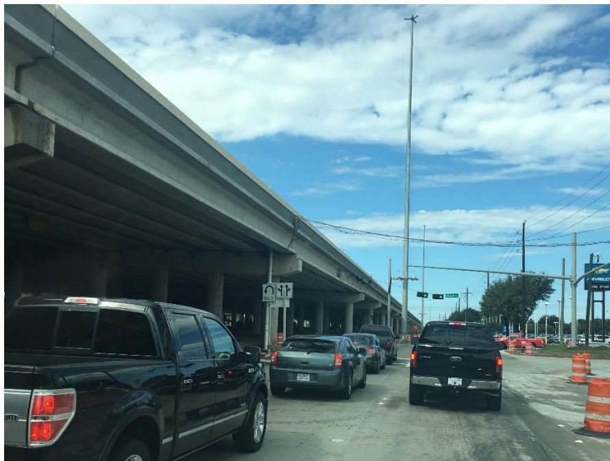
Figure 3. WB US 290 Service Road Approach
