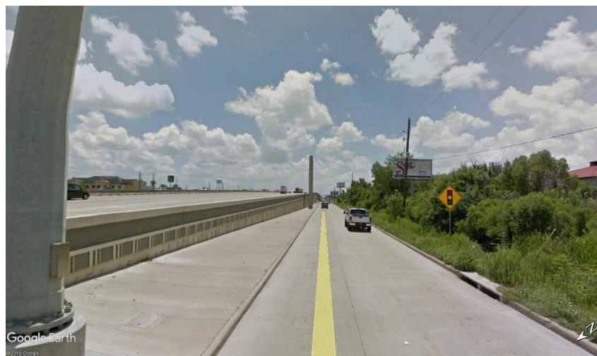
Figure 7. EB US 290 Service Road
