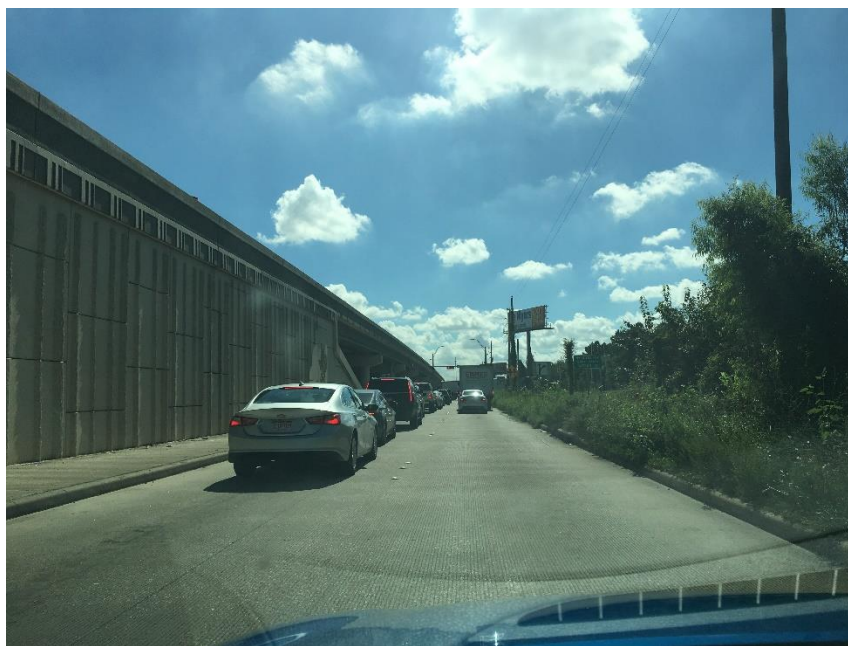
Figure 6. EB US 290 Service Road Approach
