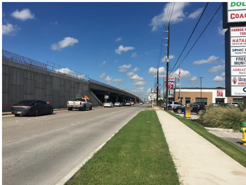
Figure 3. WB US 290 Service Road Approach
