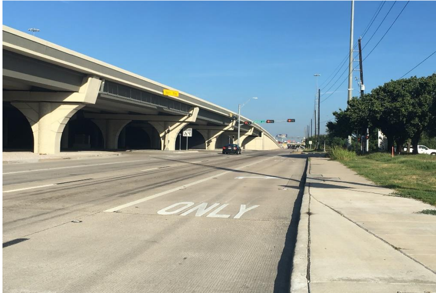
Figure 3. WB US 290 Service Road Approach
