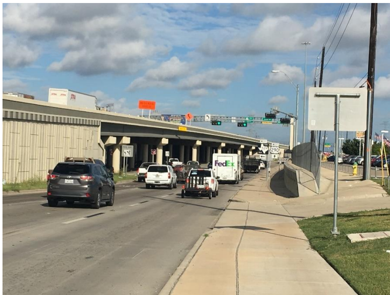
Figure 3. WB US 290 Service Road Approach
