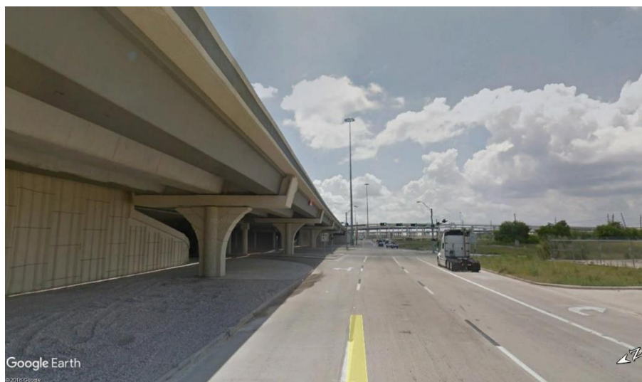
Figure 5. EB US 290 Service Road Approach
